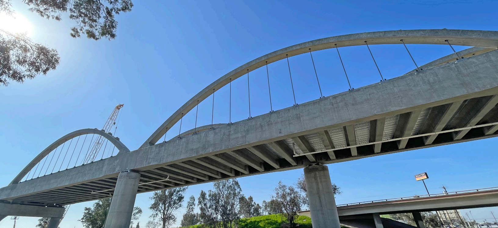
Photo: Cedar Viaduct
